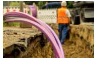
12 to 14 bar: Cable blowing and drilling
