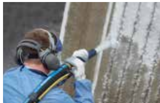
8.6 to 10 bar: Abrasive blasting
